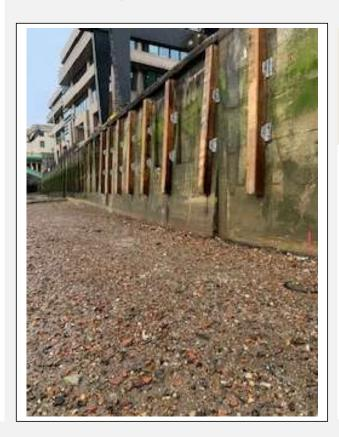
Campshed reprofiled, along with installation of new 'Greenheart' vertical timber fenders
