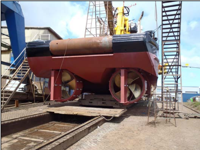
View on stern after fitting Props, and rudders 12-7-2017
